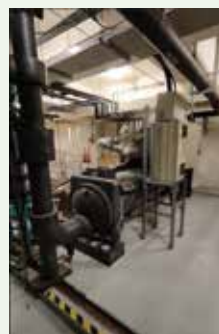
Headquarters VFD on Chillers Installation
